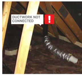
EXI DUCT TOO LONG AND NOT SUPPORTED = FANS WILL BE NOISY / INEFFICIENT. VENTILATION COMMISSIONING NOT DONE CORRECTLY
